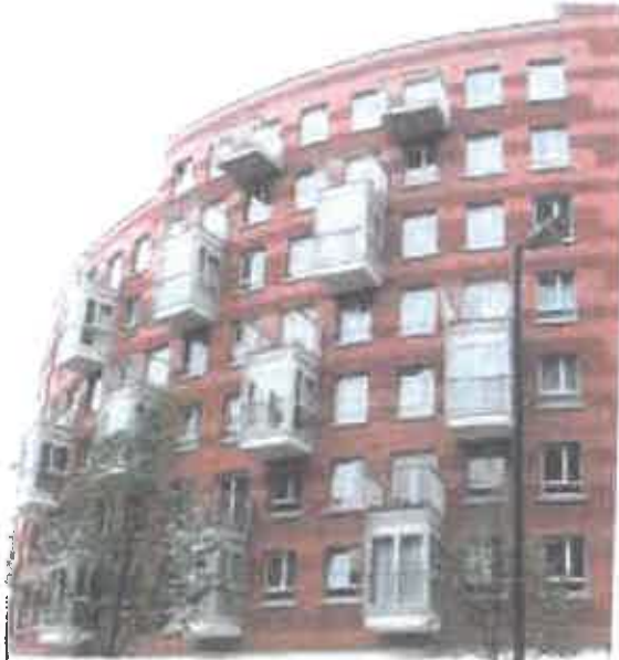
Figure 2.1. Old North London characteristc architecture. (VSC) by computer calculations to measure daylight to be brought in. Where a balcony is above a living room the relevant measurement is taken from an adjacent ground floor window.
